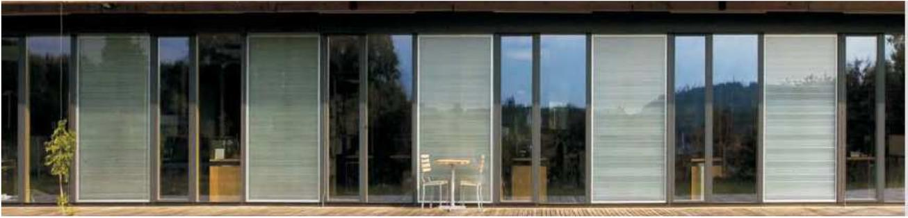
Figure 28: Windows with PCMs integrated in their panes (the translucent ones). Courtesy of GlassX.
