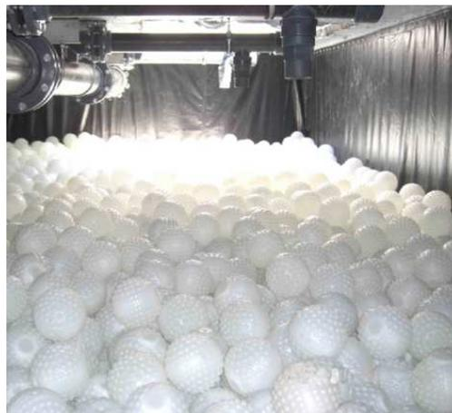
Figure 27: Ice capsules for ice thermal storage in an air conditioning installation. Cryogel.
