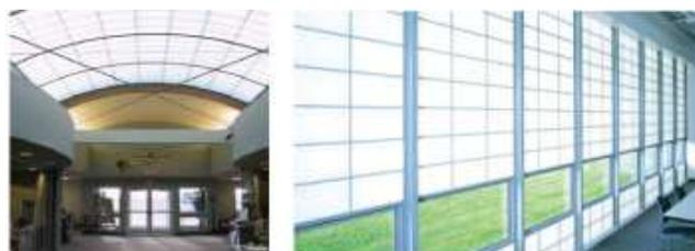
Figure 12: Two applications of panels filled with granular aerogel (Xtralite and Lumira).
