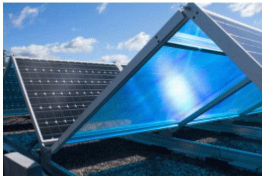
Figure 18: Reflectors between two rows of solar panels (courtesy of <http://www.f2e.es>).
