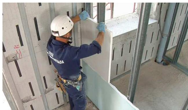
Figure 26: Energain panels being installed.
