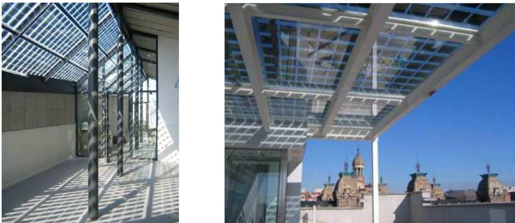
Figure 14: Two examples of the use of solar cell glazing. Extracted from VidurSolar Brochure.
